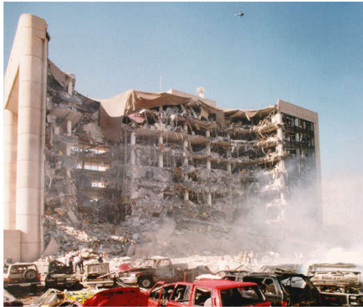
Fig 1.2. The Alfred P. Murrah building in Oklahoma
