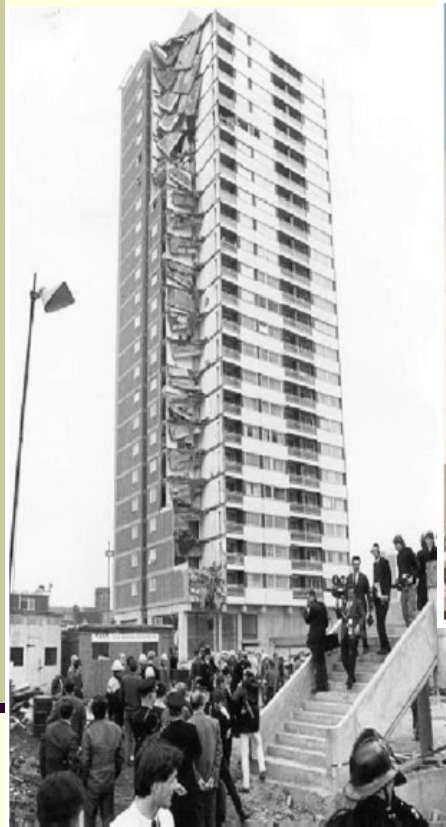
Fig 1.1. The Ronan Point apartment building
