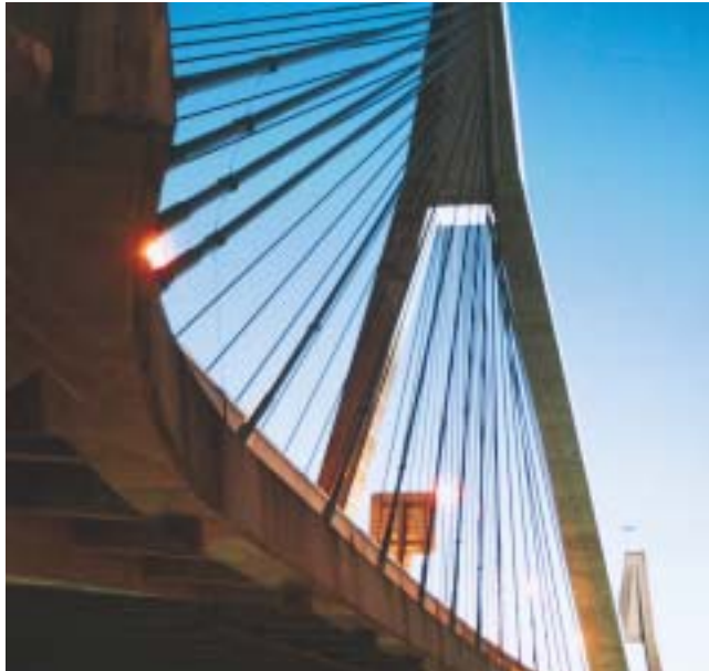
Whilst this sign on the Anzac Bridge is necessary the photograph shows how the sign interferes with the aesthetics of the bridge.
