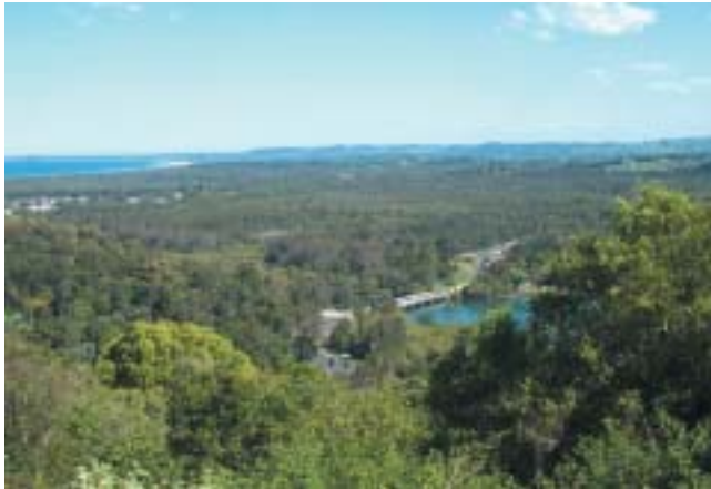
The structure of the bridge over the Brunswick River at Brunswick Heads is not visible from the Pacific Highway, yet it forms a small but significant part of the landscape when seen from a local scenic viewpoint.
