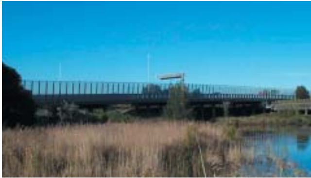
Acrylic panels on the M5 East maintain the slenderness of the bridge structure whilst minimising the dominance of the structure on surrounding areas.
