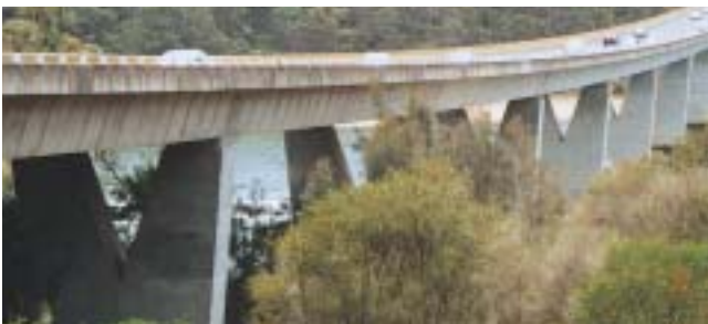
The bridge over Georges River.
