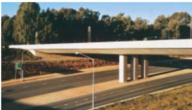
Overbridge in Canberra. The continuous, clean lines of the parapet, which continue past the abutment, help visually anchor the bridge in the landscape.
