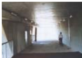
Footpath connection under the bridge.
