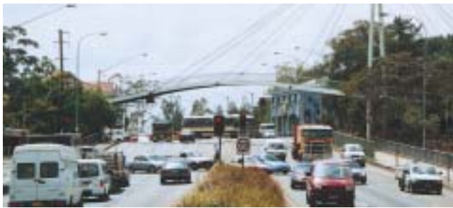
Cable stay bridge over Pennant Hills Road.
