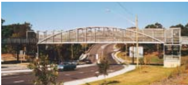
Steel truss bridge over Bexley Road.
