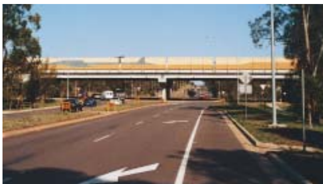
A simple pier and girder bridge, which without the noise walls may have appeared more slender. The visual slenderness ratio is approximately 1:6.
