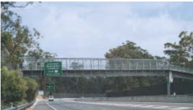
The ramp and bridge connection on this pedestrian bridge is seamless, note the attention to detail of the narrowing of the edge of the deck as it passes over the thicker section of girder above the pier.
