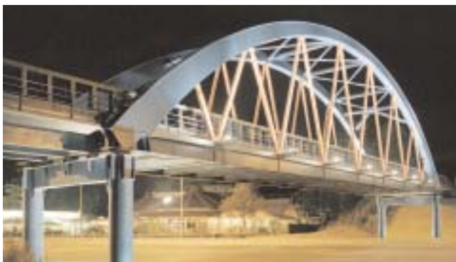
Rail bridge over the highway at Coffs Harbour.
