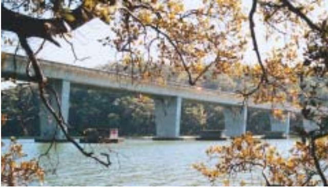
Bridge over the Georges River at Alford's Point. The minimal profile maximises views of the landscape.
