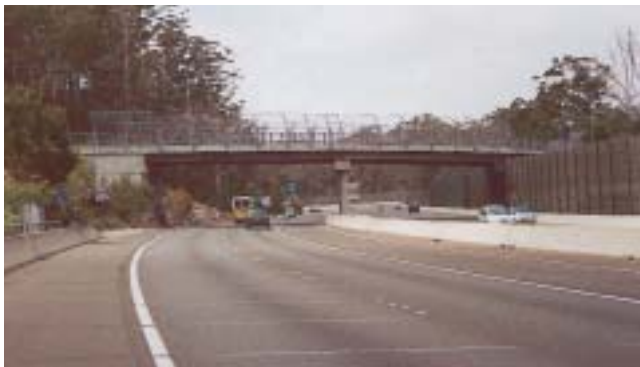
Bridges over the F6 and M2 Infilled abutments are often dominating structural elements with little aesthetic merit especially in a landscape setting. If possible, they should be avoided or eliminated in the design process.
