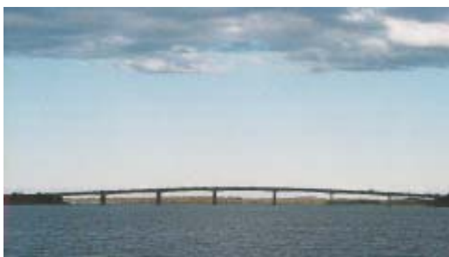
Captain Cook bridge, a slenderness ratio of approximately 1:18.
