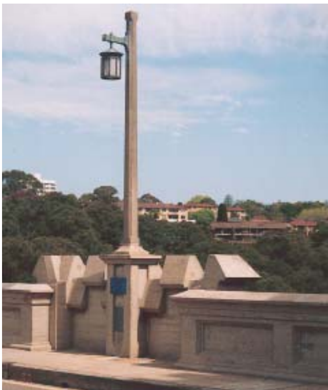
The attention to detail on the 1939 upgrade of the suspension bridge at Northbridge is exemplary.
