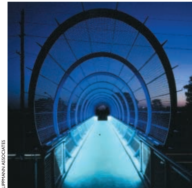
Pedestrian bridge over the Horsley Drive in Fairfield. The safety screen totally surrounds the walkway however the oval shape softens the cage effect. The user experience would be interesting both day and night.
