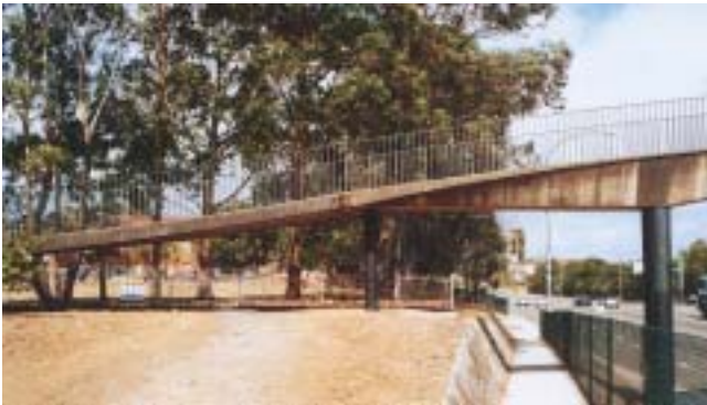
The ramp and bridge connection on this pedestrian bridge is seamless, note the attention to detail of the narrowing of the edge of the deck as it passes over the thicker section of girder above the pier.
