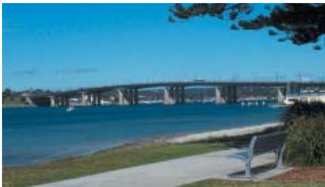
Graceful pier spacings on Captain Cook Bridge over the Georges River.
