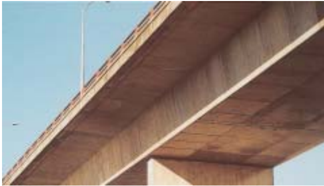
The proportions of elements in the cross section of a bridge are an important aesthetic consideration. (Bridge over the Hunter River at Stockton).
