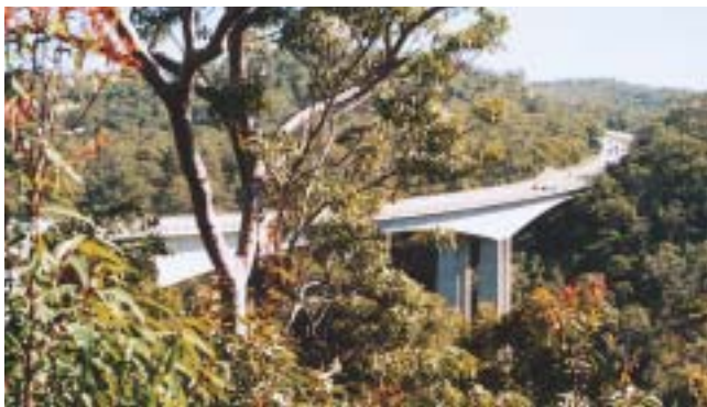
The simple uncluttered shape of the twin bridges over Mooney Mooney Creek does not detract from the natural bushland of the Hawkesbury valley.
