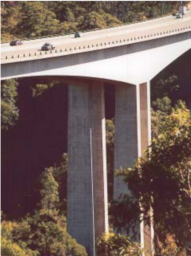
Multiple piers both along the bridge and across the bridge can be a significant feature of a bridge and if well designed can provide character and great strength. (Twin bridges over the Mooney Mooney Creek).
