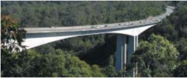
Haunched girders on the twin bridges over Mooney Mooney Creek, NSW.
