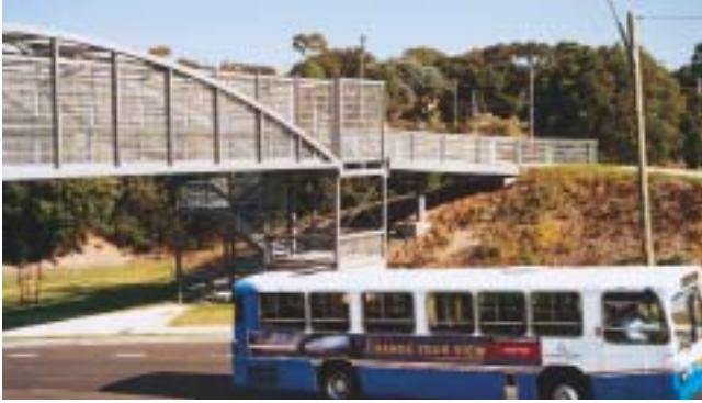
Bridge over Bexley Road. The gradient of the access ramp can be minor if the road is on a slope.
