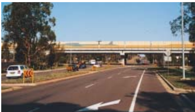
Noise Walls on the bridge on the Pacific Highway near Raymond Terrace also add to the perception that the bridge is less slender than it is.
