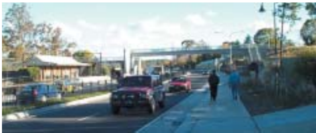
Haunched concrete feature bridge over the Great Western Highway, Falconbridge.
