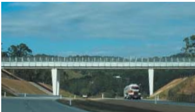
Bridge over the Pacific Highway on the Yelgun to Chinderah upgrade. The reverse taper appears refined and well detailed. It creates an impression of strength and solidity between pier and superstructure and eliminates the need for a headstock.
