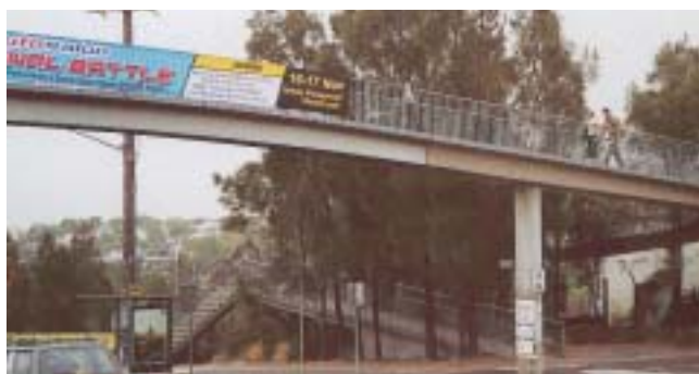
The ramp on this bridge over Victoria Road in Rozelle is well integrated with planting and provides an interesting user experience walking up into the canopy of the Casuarinas.
