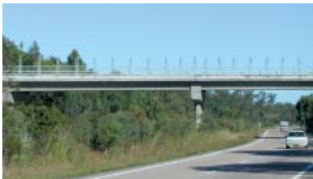
An overbridge with a slenderness ratio of approximately 1:12.
