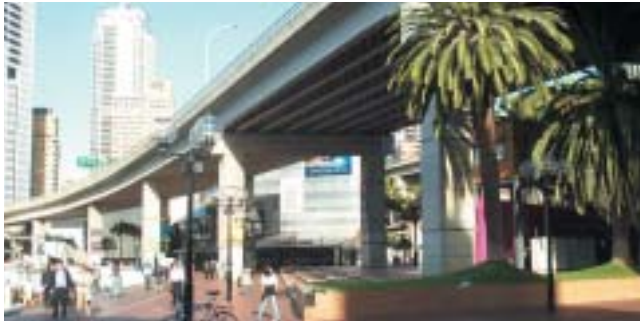
The pier and headstock combination on this bridge over Darling Harbour provides a reassuring impression of strength as well as a high degree of permeability for light and pedestrian movement.
