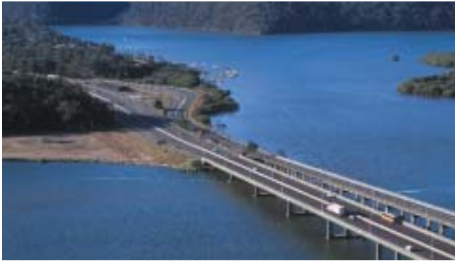
The bridges over the Hawkesbury River at Brooklyn. The proximity of these bridges results in an interplay between the designs. The two bridges are not separate but seen as one visual entity.
