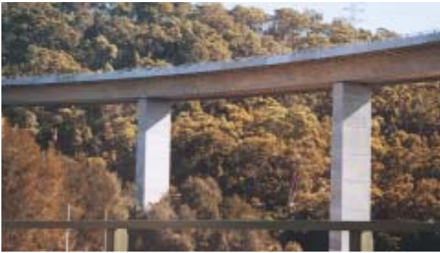
Bridge over the Woronora River at Alford's Point. The minimal profile maximises views of the landscape.
