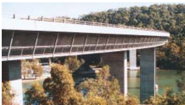
The slung footpath on the bridge over the Woronora River allows dramatic views of the valley. A widened viewing area in the middle of the bridge allows pedestrians to stop and appreciate the structure in its setting.
