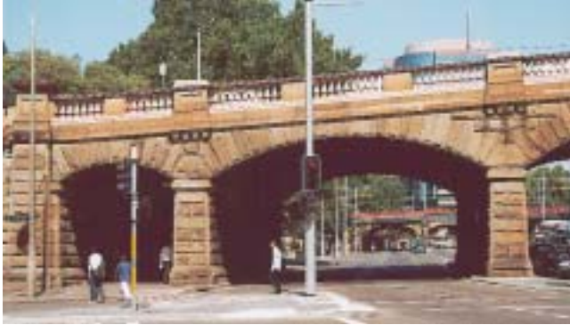
Bridge over Eddy Avenue, Central Station, Sydney. The slight taper on the abutment and piers adds character and responsiveness to the bridge and makes a more pleasant pedestrian experience.
