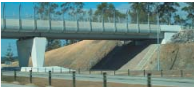
Yelgun to Chinderah, Pacific Highway upgrade.
