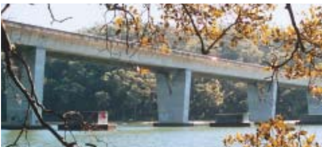
The bridge over the Georges River at Alford's Point also displays a taper although with the addition of an open pier.
