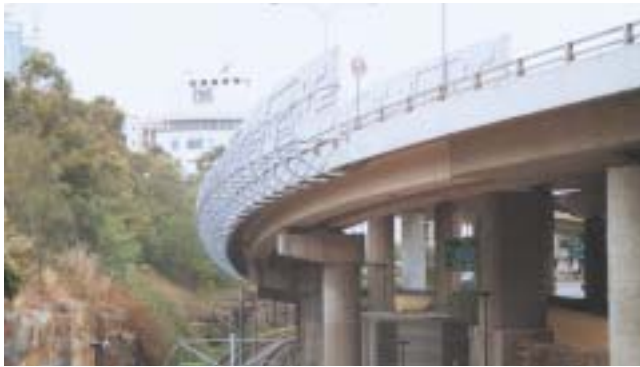
Noise walls designed to integrate with the bridge structure (Fishmarkets, Sydney).
