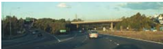
These bridges over the M4 demonstrate the impact of signage and how avoiding signs is the best aesthetic policy.
