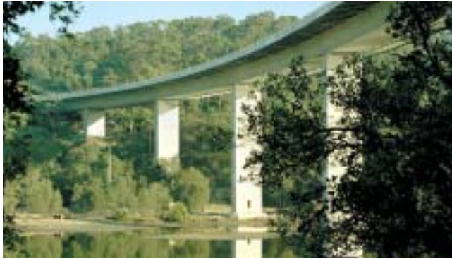
Bridge over Woronora River at Sutherland. The line of the parapet is an important bridge element. It is sharp, smooth, catches the light, helps provide shadow and unifies the structure.
