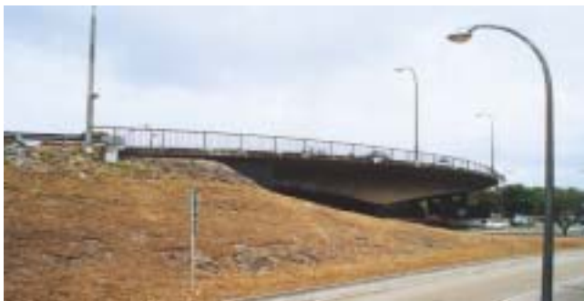
On this bridge on Victoria Road at Huntleys Point lighting is not integrated with an otherwise well designed bridge (note the tapered beam and the deep shadow line). The already complex junction between bridge barrier and safety fence needs careful consideration of details if a light column is to be included as well.
