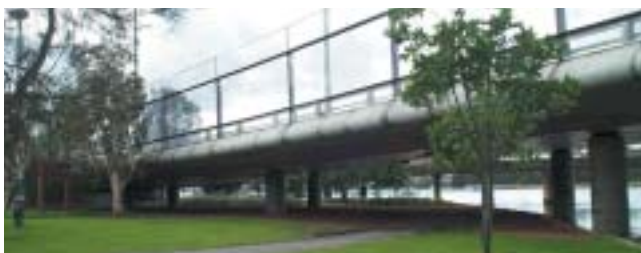
Bridge on the City West Link. A smooth curved soffit on this low bridge and pedestrian underpass helps create a pleasant environment. Note the transparent noise walls and consider the same view if the noise walls had been solid.
