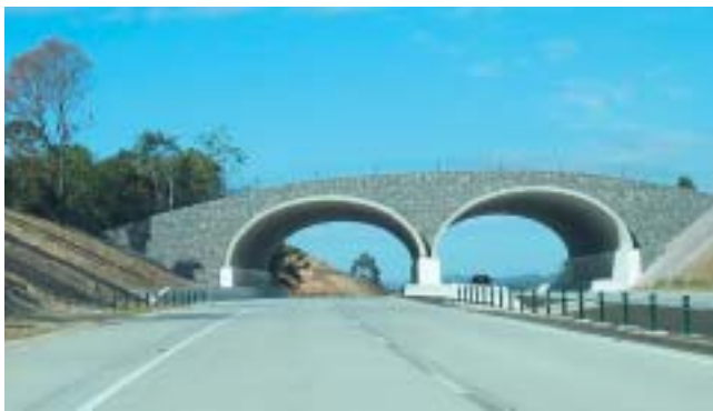
Designing the bridge so that planting is located on the bridge structure itself, further integrates nature and structure. This bridge on the Pacific Highway, Yelgun to Chinderah upgrade provides a wildlife connection and will ultimately have a visible vegetation cover on the deck.
