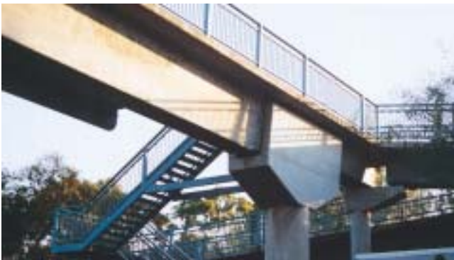
A simple connection between ramp and bridge is not achieved on these pedestrian bridges.
