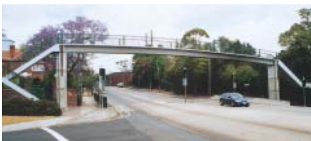
Simple beam bridge over the Pacific Highway, Sydney.
