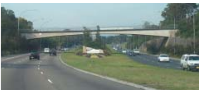
Haunched girder on bridge over Taren Point Road. It is unfortunate that the planting design is not integrated with the bridge design and obscures the fact that the bridge is a single span.
