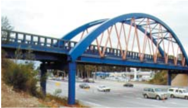
The primary colours on this rail bridge over the Pacific Highway at Coffs Harbour help create a distinctive bridge and route landmark.
