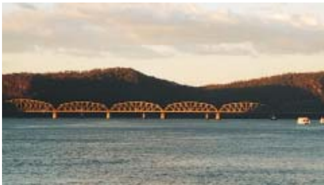
The horizontal and symmetrical nature of the rail bridge over the Hawkesbury River complements the landscape. (The oddly positioned piers in the background are remnants from an old bridge).
