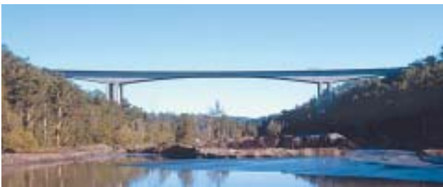
Three span haunched girder on the twin bridges over Mooney Mooney Creek, NSW.
