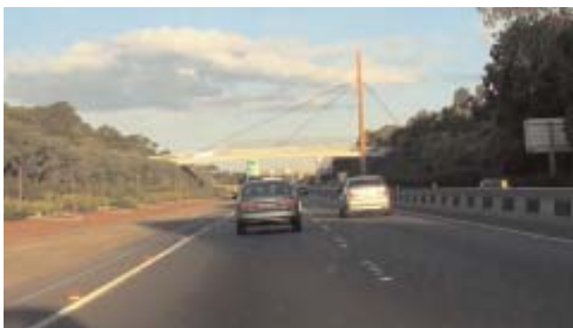
Landmark pedestrian bridge over the M4, Sydney.
