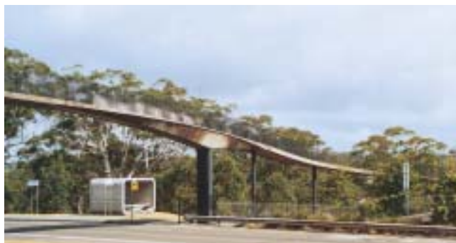
The simple spiral connection of the ramp adds to the value of the bridge. However adequate space is required for this solution.
