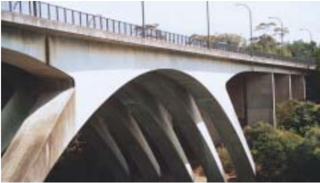
Multiple piers on the bridge over the Tarban Creek are visually distinctive and help create a strong sculptural effect.
