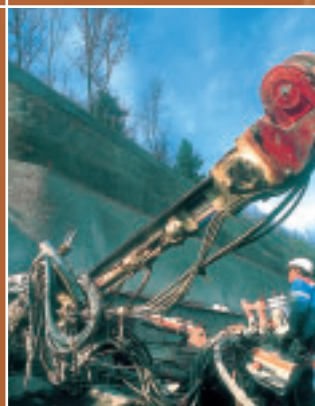
◀ PRESTRESSED GROUND ANCHORS
