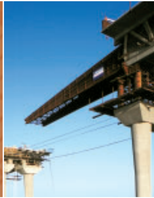
◀ LAUNCHING FRONT NOSE ASSEMBLY
