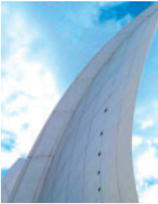
◀ PRESTRESSING OF PRECAST ELEMENTS
