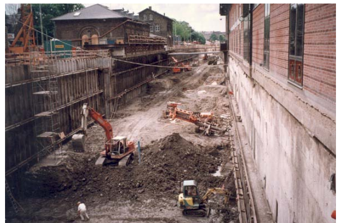
Figure 1. Overview of the drilled-pile wall at Fredriksberg Station, Copenhagen
