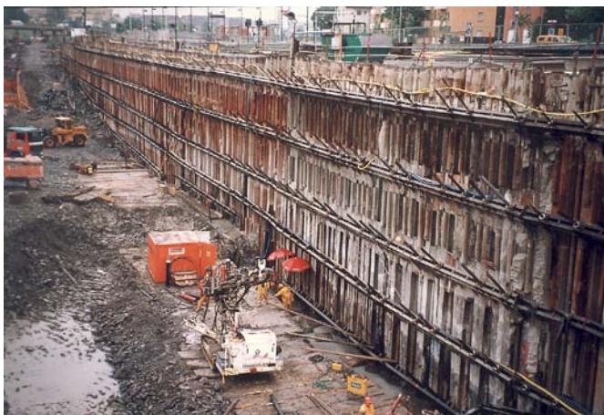
Figure 4. Overview of sheet pile wall at project SL-10, South Link, Stockholm
